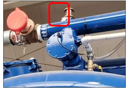
Figure 18: Media Filter Sight Glass
