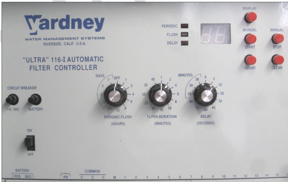
Figure 68: Automatic Filter Controller
