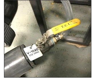
Figure 9: EC Drain Valve
