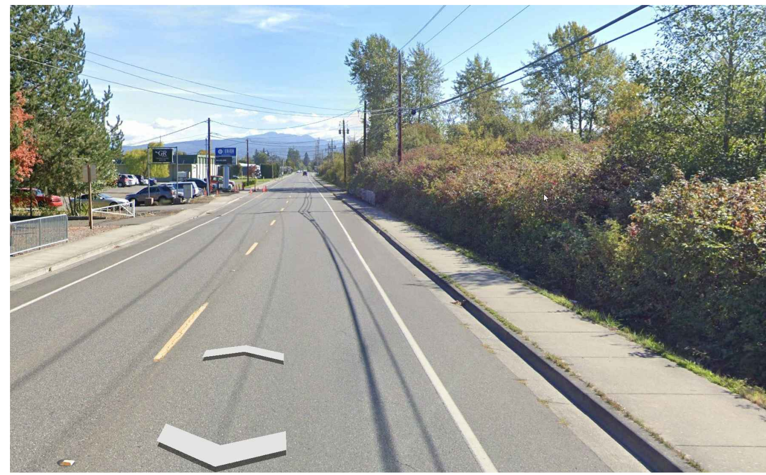
STREET VIEW LOOKING SOUTH (NORTH OF EXISTING DRIVEWAY ENTRANCE)
