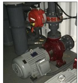
Figure 3: EC Supply Pump
