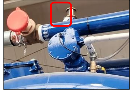
Figure 18: Media Filter Sight Glass
