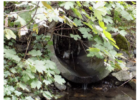
Marine Drive Outfall
