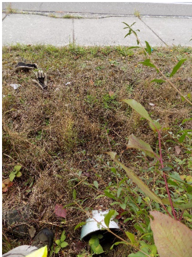
Marine Drive Open Channel
