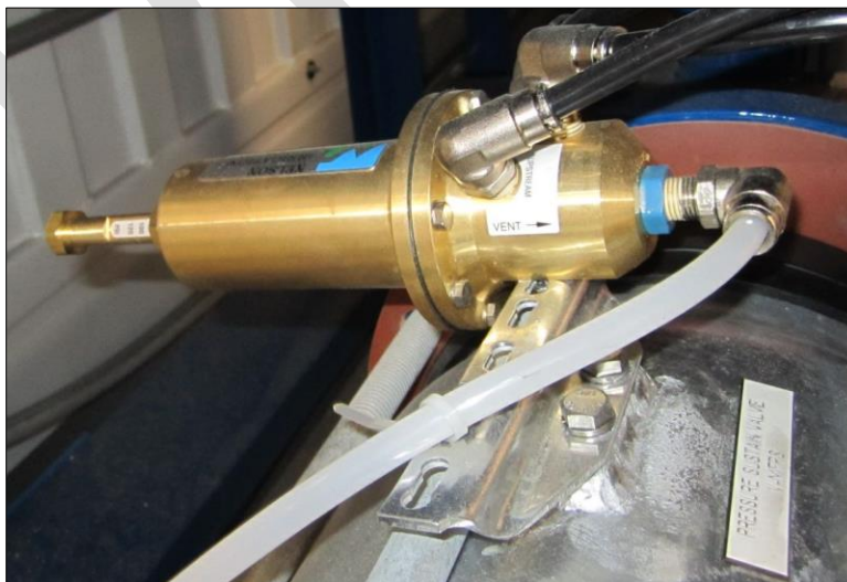
Figure 67: Pressure Sustaining Valve
