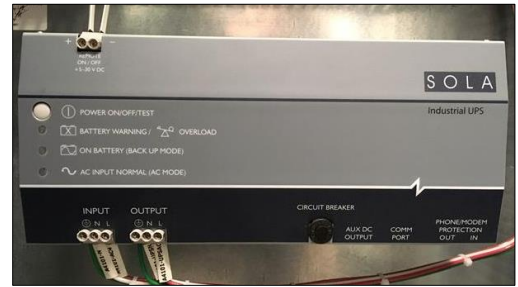
Figure 34: Uninterruptable Power Supply
