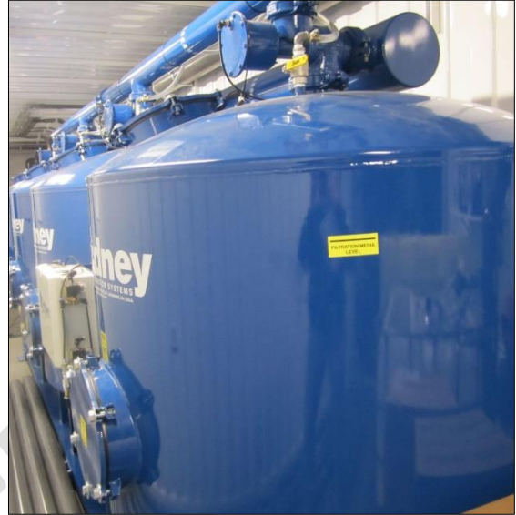
Figure 1: Example Media Filter
