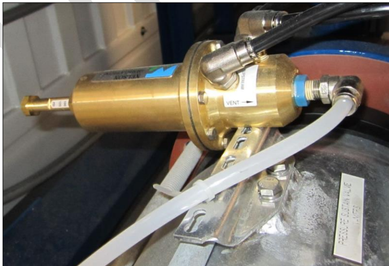
Figure 67: Pressure Sustaining Valve
