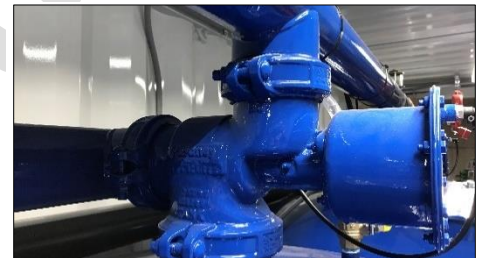
Figure 16: Three-Way Valve
