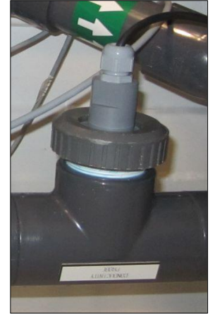
Figure 28: Conductivity Probe
